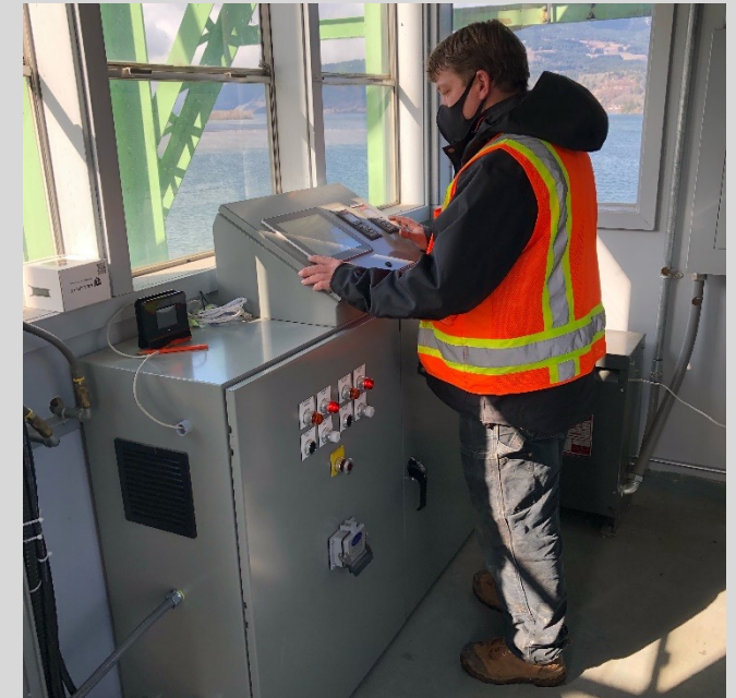
2019 Skew System & Span Drive Motor Rehabilitation
