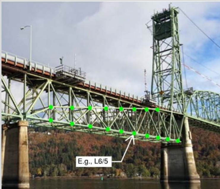
2017 Auxiliary Truss Repairs
