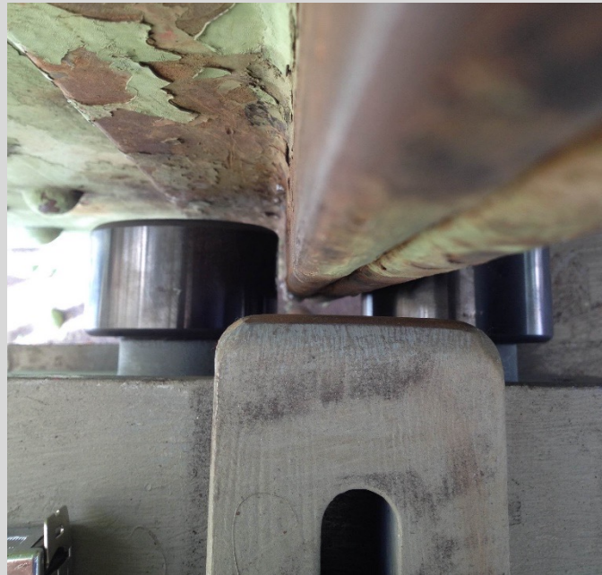
2016 Span Guide Replacement & Repairs
