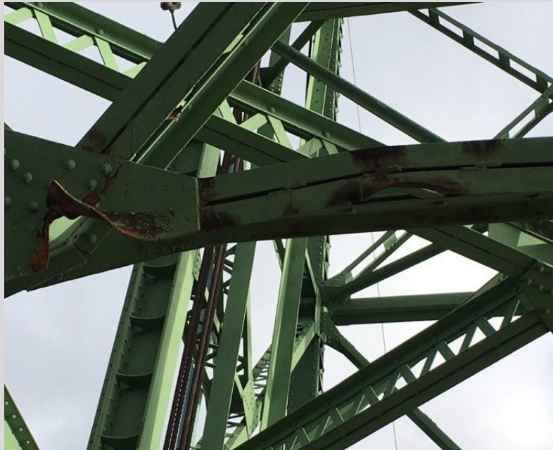
2019 Portal Truss Repair
