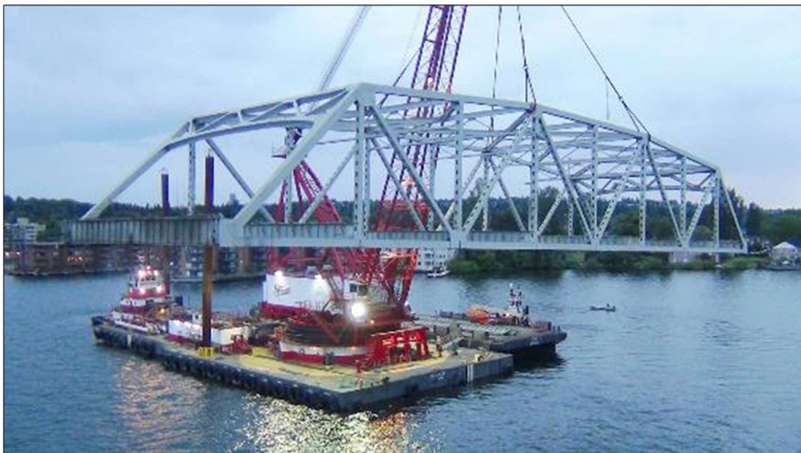
Image 6. Removal of the 1963 Floating Bride Truss on FB&L Project
