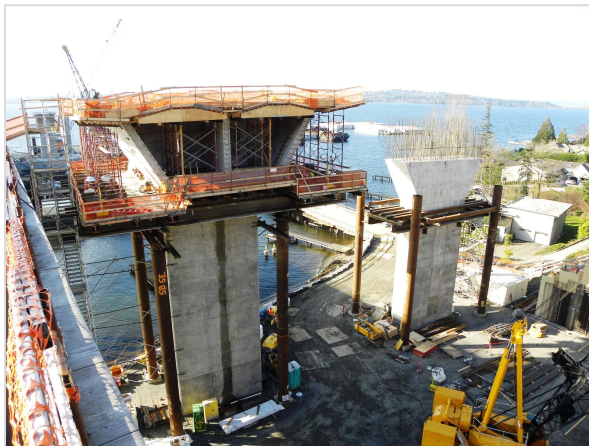
Image 1. Pier Segment and Form-Travelers
