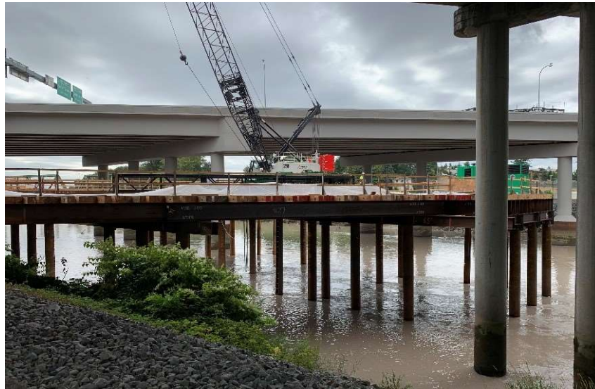
Image 6. Work Trestle Configuration in Puyallup River
