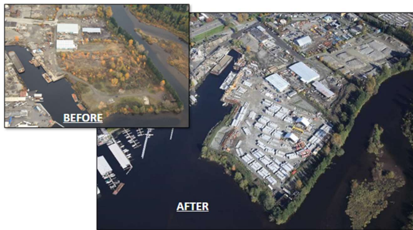
Image 5. Site Access for WSDOT SR 520 FB&L Project
