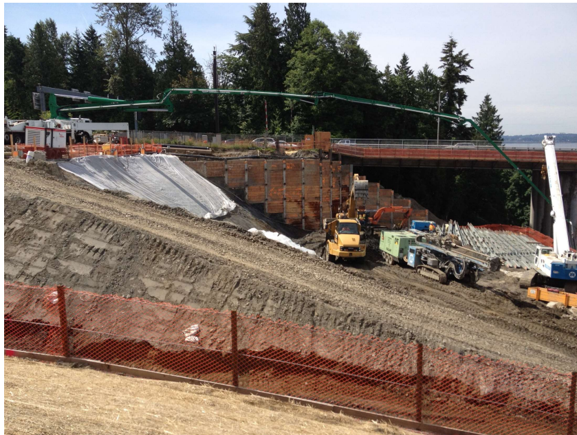
Image 4. Steep Access Down to Water at FB&L Project
