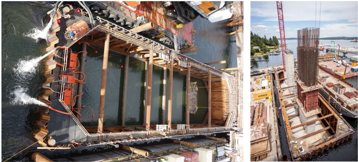
Image 7. Cofferdam Images at FB&L Project
