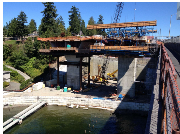
Image 1. Pier Segment and Form-Travelers
