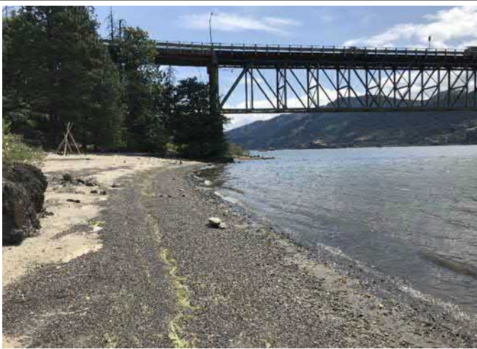
Photo 1. Nearshore and OHHM conditions on WA side, facing East
