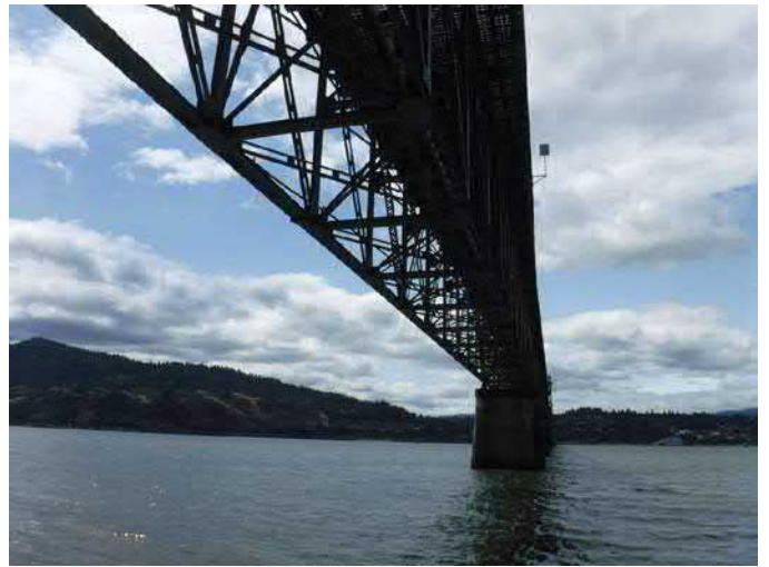
Photo 4. Existing bridge facing south from WA side
